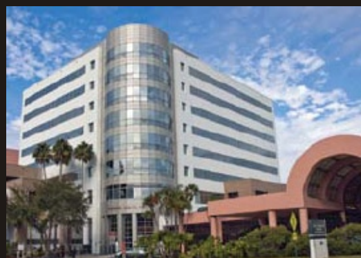
WALDEMERE MEDICAL PLAZA RENOVATIONS
