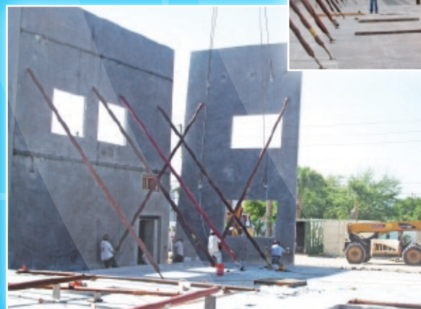
Erection of Concrete Tilt Panel Walls MAY 13
