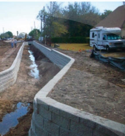
Earthwork Underway MARCH 10
