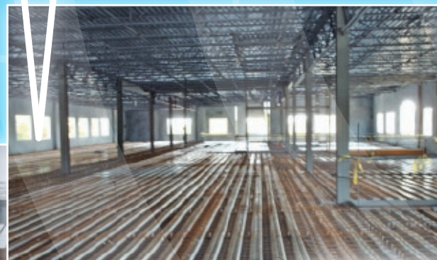
2nd Floor Metal Decking JUNE 11
