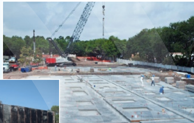
Concrete Slab and Tilt Panels MAY 5
