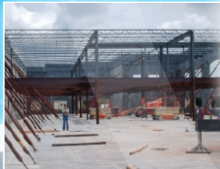
Structural Steel Framing MAY 19
