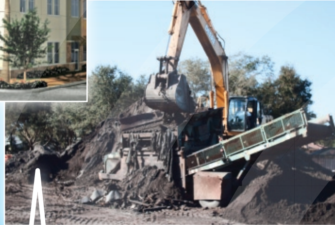
Apartment Demolition by Sonny Glasbrenner FEBRUARY 10
