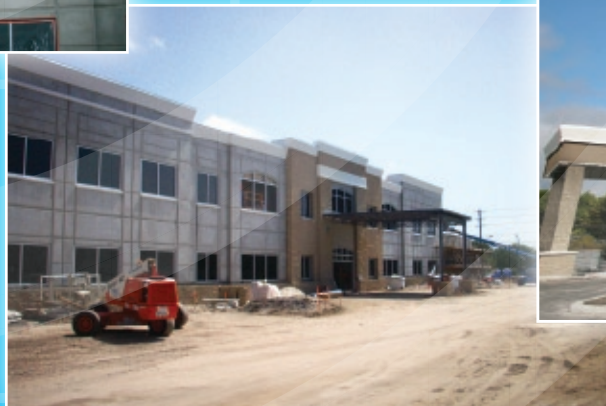
Painting and Masonry Veneer JULY 14
