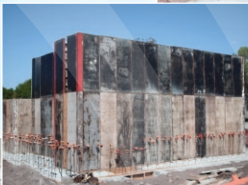
Forming of PET/CT Scanner Vault Walls APRIL 9
