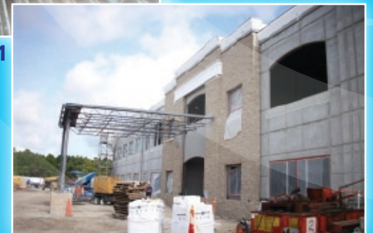
Roofing Work Underway JULY 14
