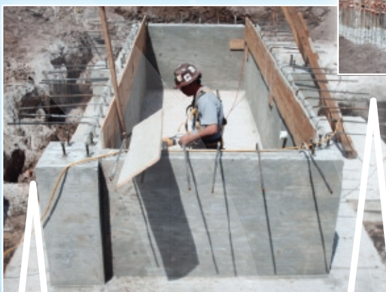
Structural Foundations MARCH 19
