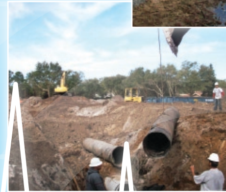
Underground Utility Installation FEBRUARY
