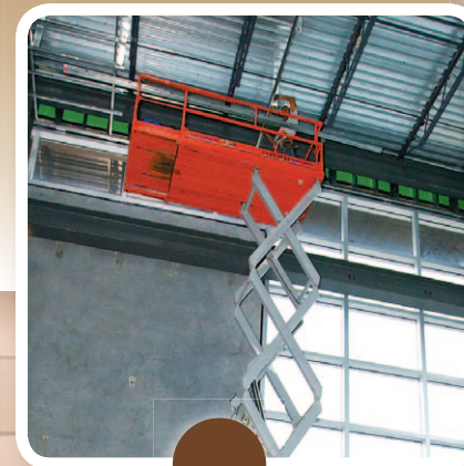
06.12.2012 Installation of sunshades and other exterior finishes
