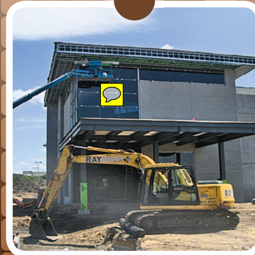
04.11.2012 Interior build out and installation of StormTec drainage system
