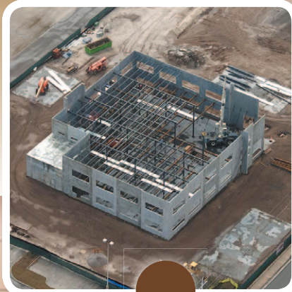
01.13.2012 Standing of tilt panels and beginning of structural steel
