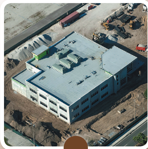
03.12.2012 Roof system completion and installation of windows
