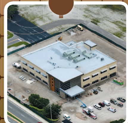
07.13.2012 Site preparation for paving
