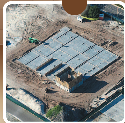
11.11.2011 Slab on grade and forming of tilt panel walls
