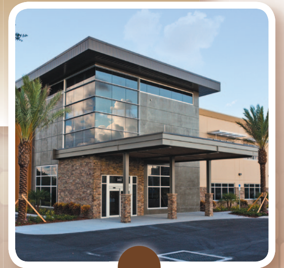
09.12.2012 Completion of paving and building systems start up and certification
