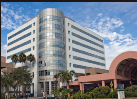
WALDEMERE MEDICAL PLAZA RENOVATIONS
